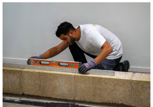
5 It is essential for this base course to be perfectly level. Check the perpendicularity and wait for the mortar to dry before continuing the masonry.
