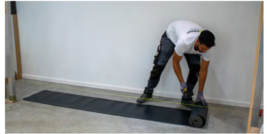
2 The IsoHemp blocks must be protected from capillary rise. Apply a sealing tape (of the DIBA type) going up a couple of cm along the IsoHemp block.
