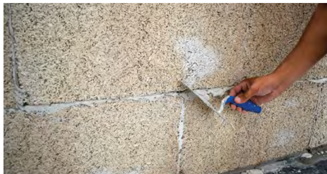
10 Remove excess adhesive using the trowel.
