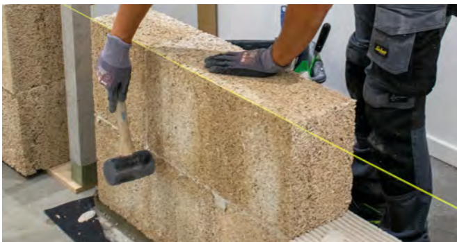
9 Adjust with a mallet and check the levels.
