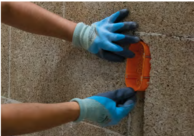
3 Fix the boxes and electrical cable ducts.
