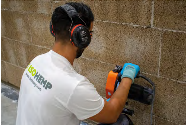
1 Create the grooves using a grooving machine.
