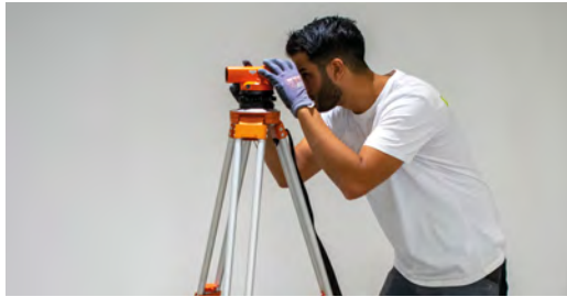
1 Find the highest point of the slab with a laser or water level.
