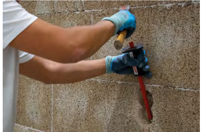
2 Finish the opening manually.
