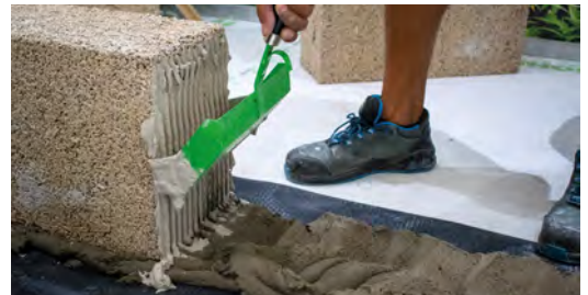
4 Glue the vertical joint (except for the blocks of 30 and 36cm with tenon and mortise joints) and lay the next block. Adjust with a mallet if necessary to obtain a 3 mm vertical slim joint.
