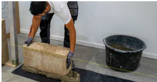
3 Apply a uniformly spread mortar bed 1 to 2 cm thick.
